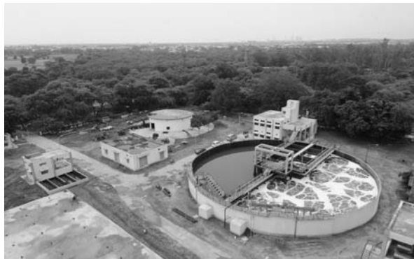
Figure - 5 : Bird's Eye view of the Recycling STP Sargasan
