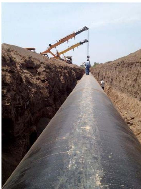
**Fig 9. Some of the first pipe lengths being installed in the Gujarat water project**
