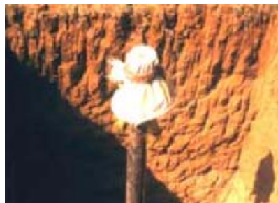
Fig 8 Making Of Borehole
