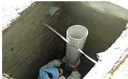
Fig 12 wrapping of perforations
