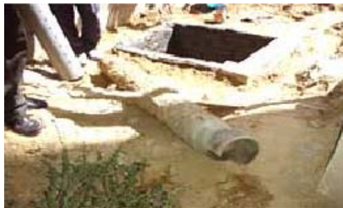
Fig 11 replacing ci pipe with perforated pvc pipe
