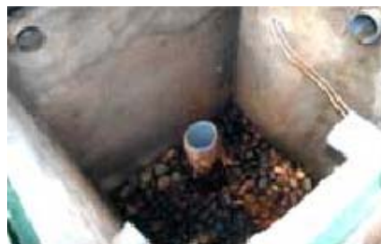
Fig 9 Providing Masonry Or RCC Walls
